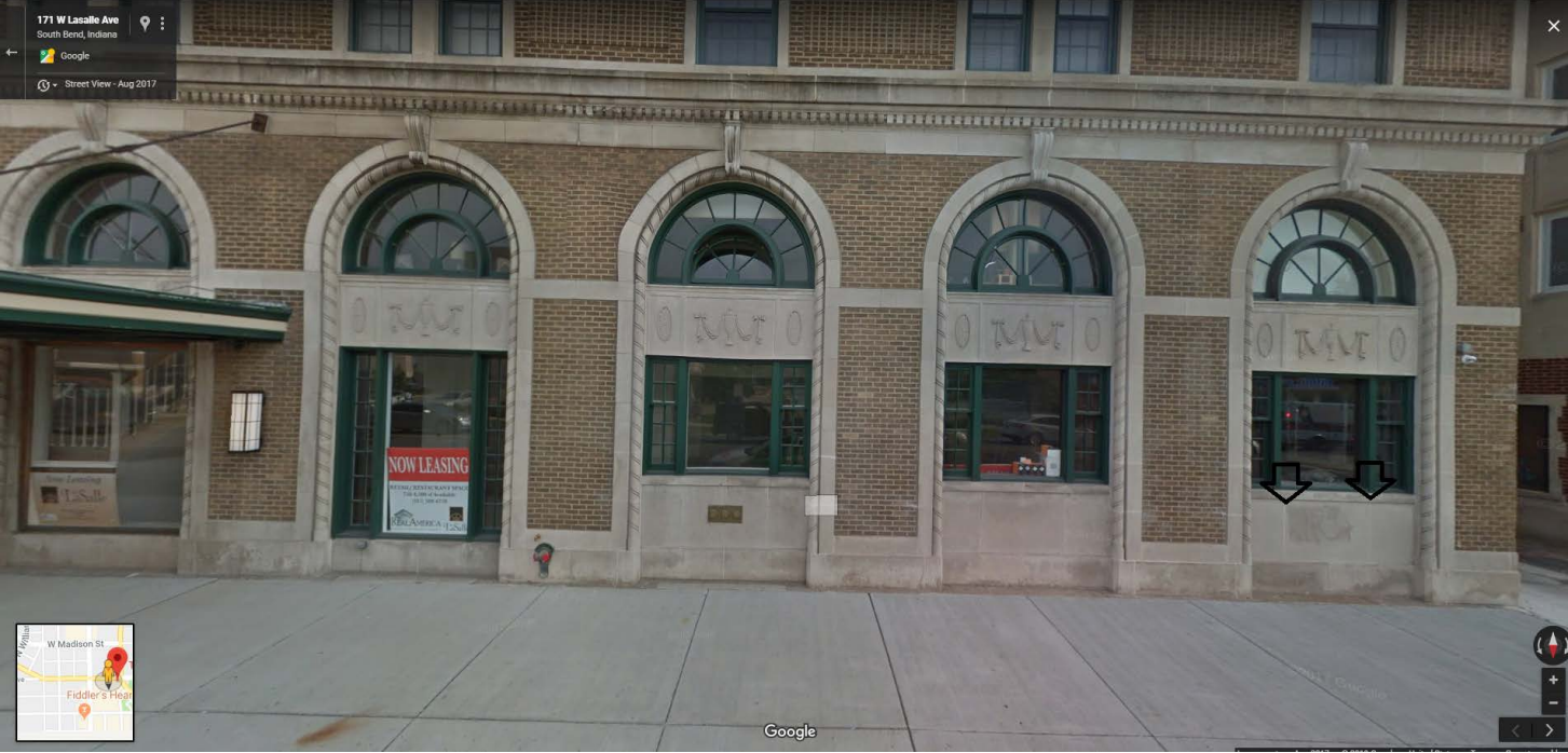
DETAIL PICTURE - Location of proposed ADA ramp and new door.
