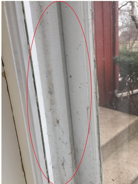
"Warped frame won't latch"
