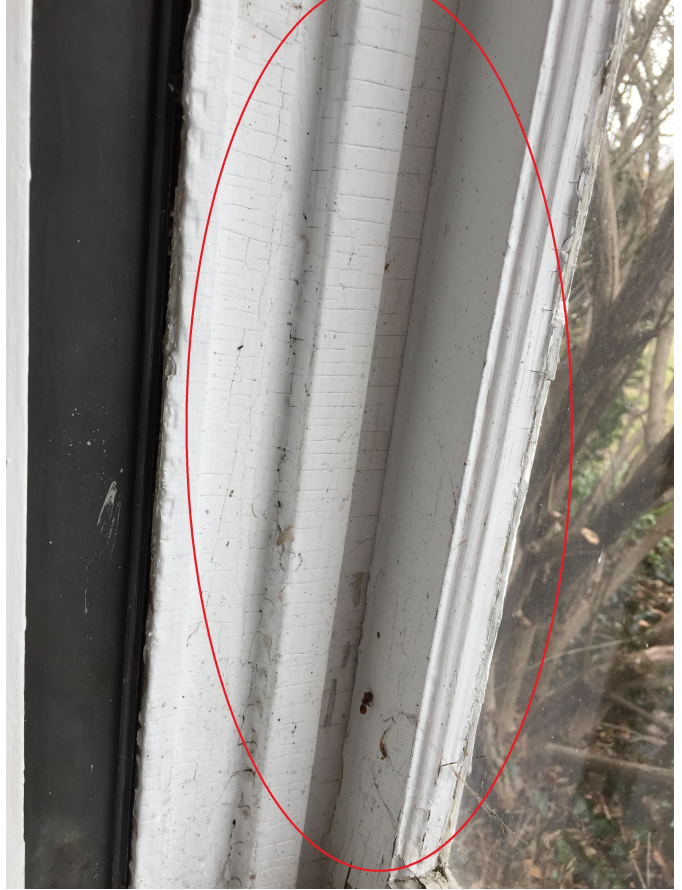
"Warped frame won't latch"
