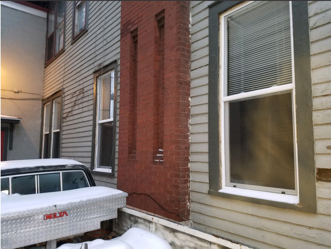
SIDE PICTURE (NORTH) - Close-up of each replaced window, taken 1/24/2019.
