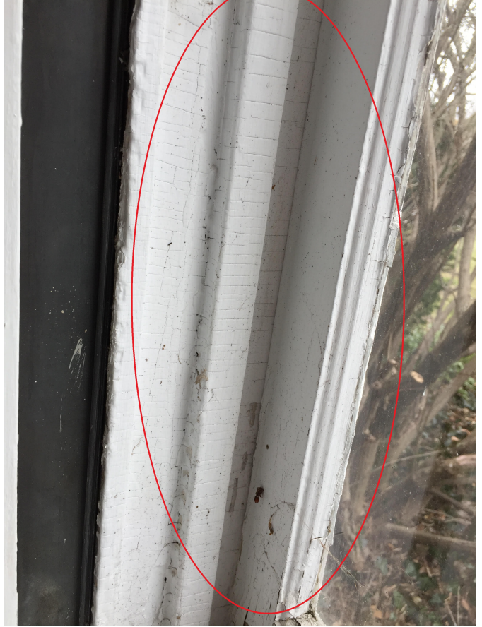
"Warped frame won't latch"
