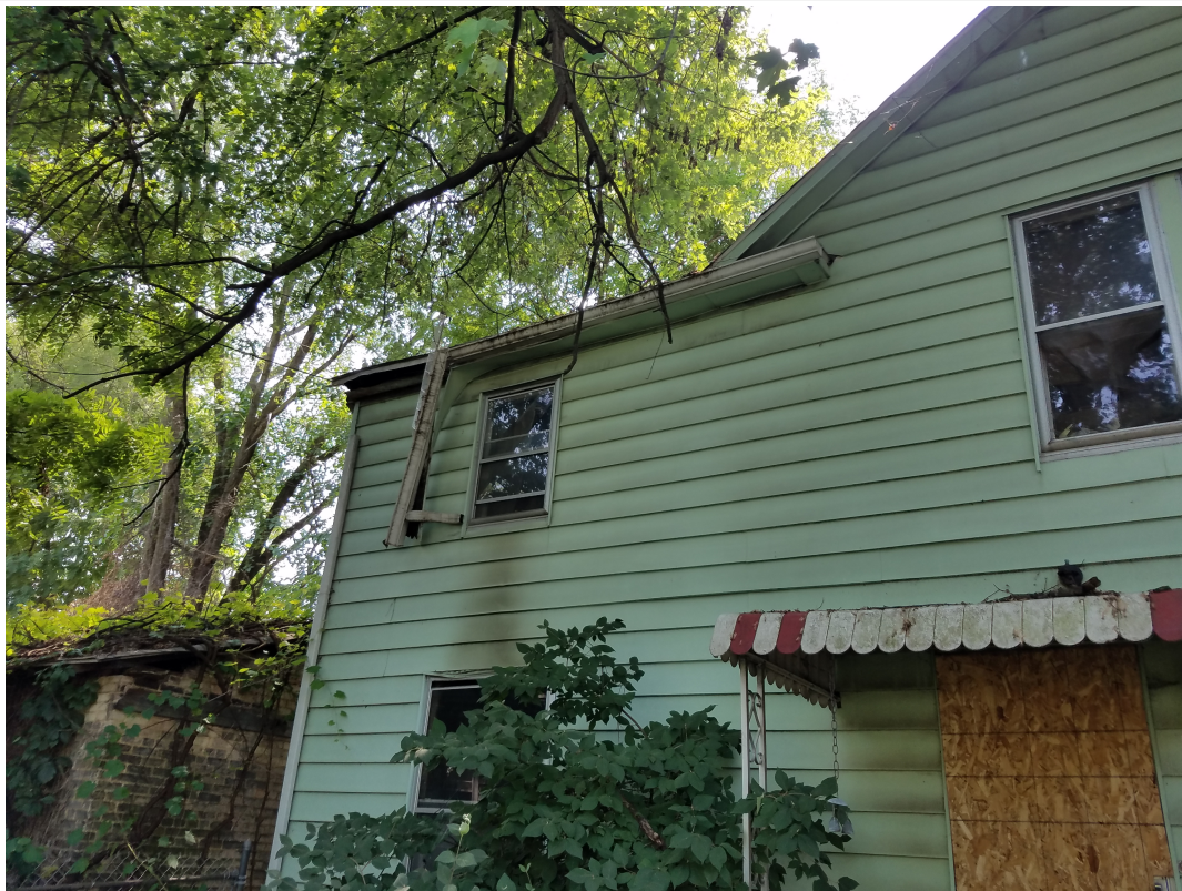
SIDE PICTURE (NORTH EAST) - Picture of the side of the building.
