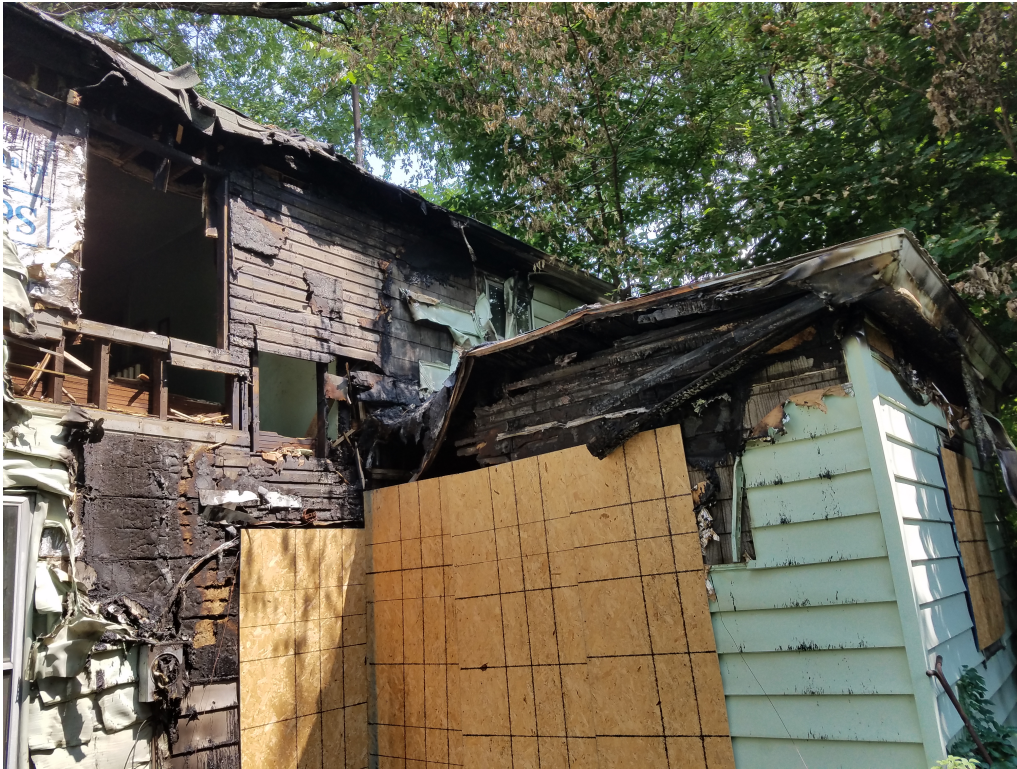
SIDE PICTURE (SOUTH EAST) - Picture of the side of the building.
