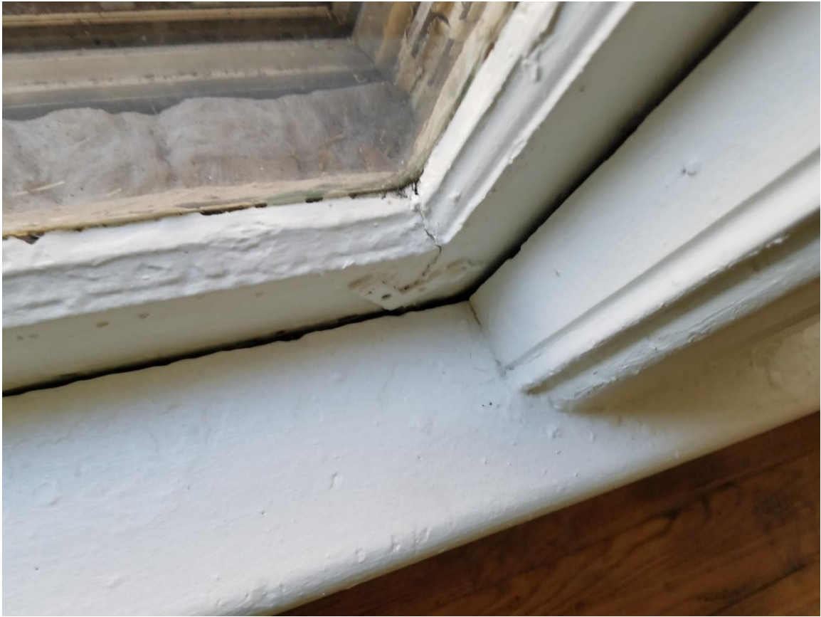
Figure 3 - lower level sill. – Photos from September.
