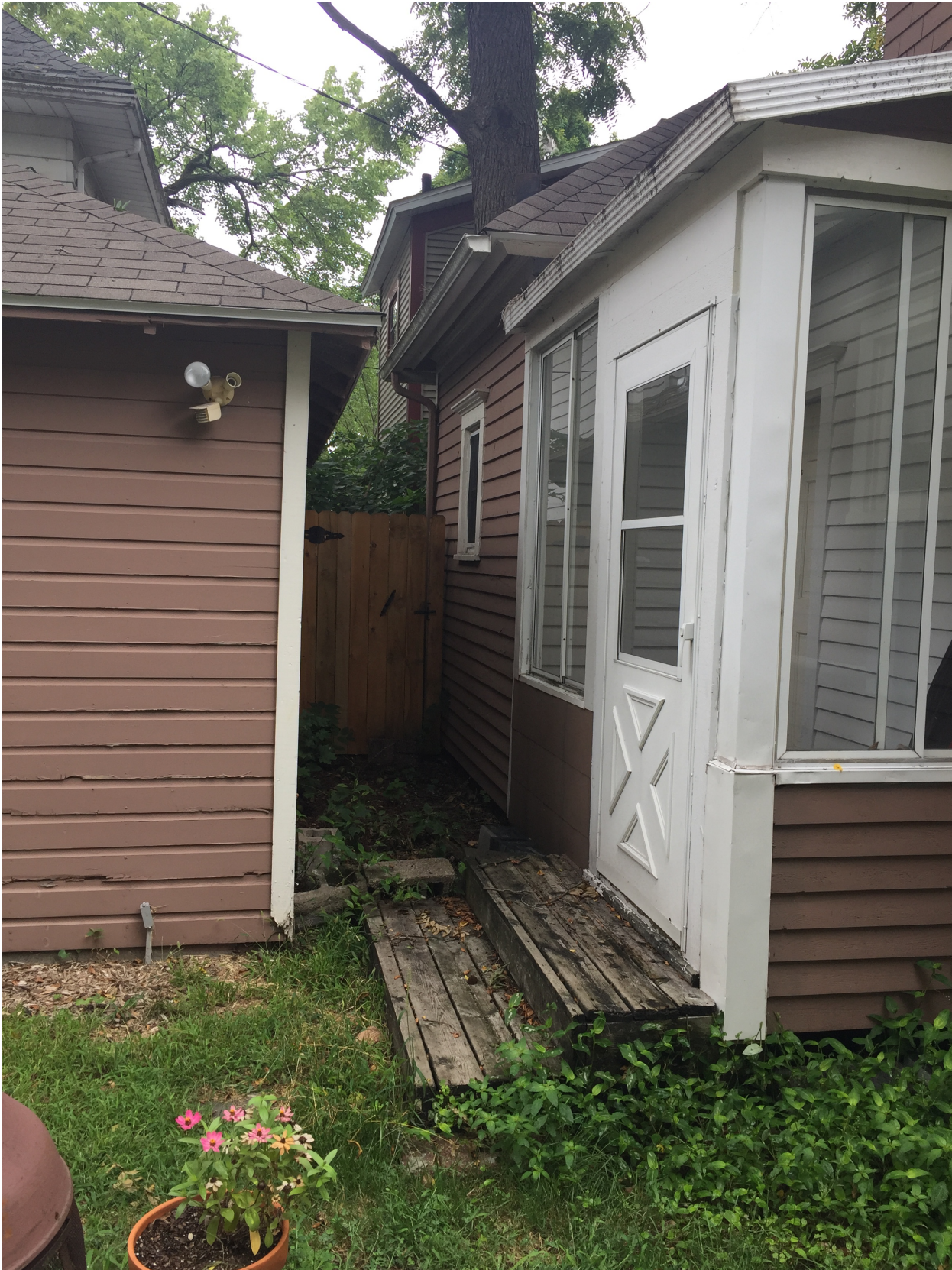
West Elevation (Side C)
