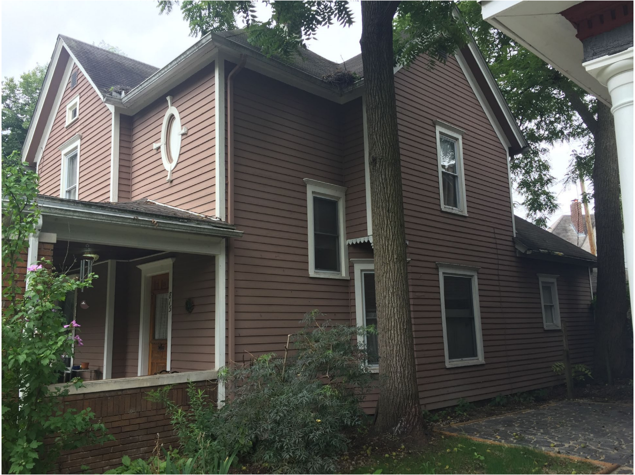
North East Elevation (Side D)
