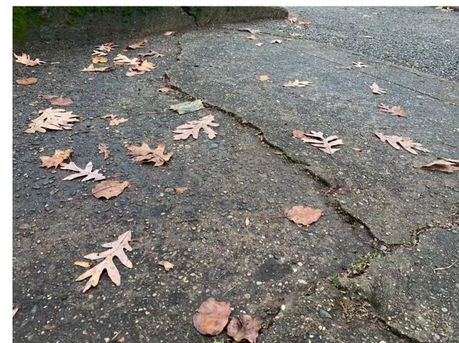
Bottom landing - multiple cracks, unevenness, ADA issue
