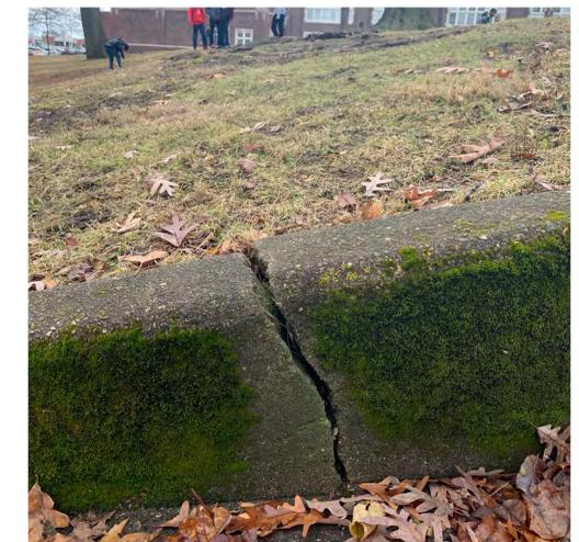
Middle landing - crack in wall, both sides
