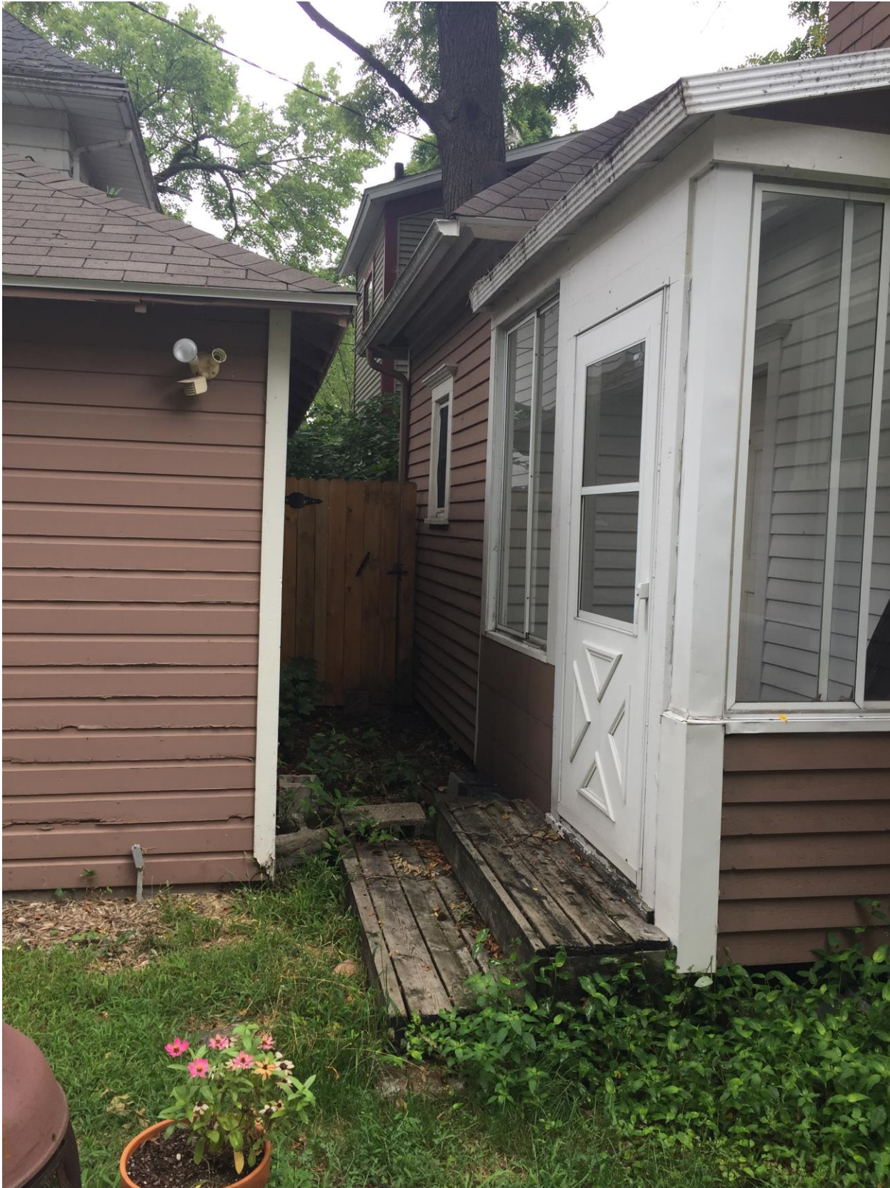
West Elevation (Side C)
