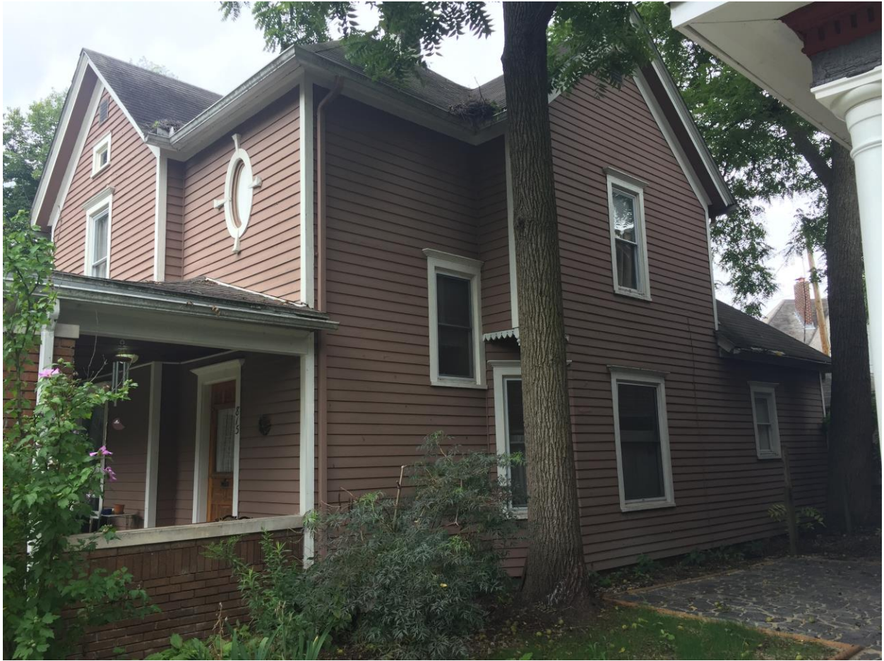
North East Elevation (Side D)
