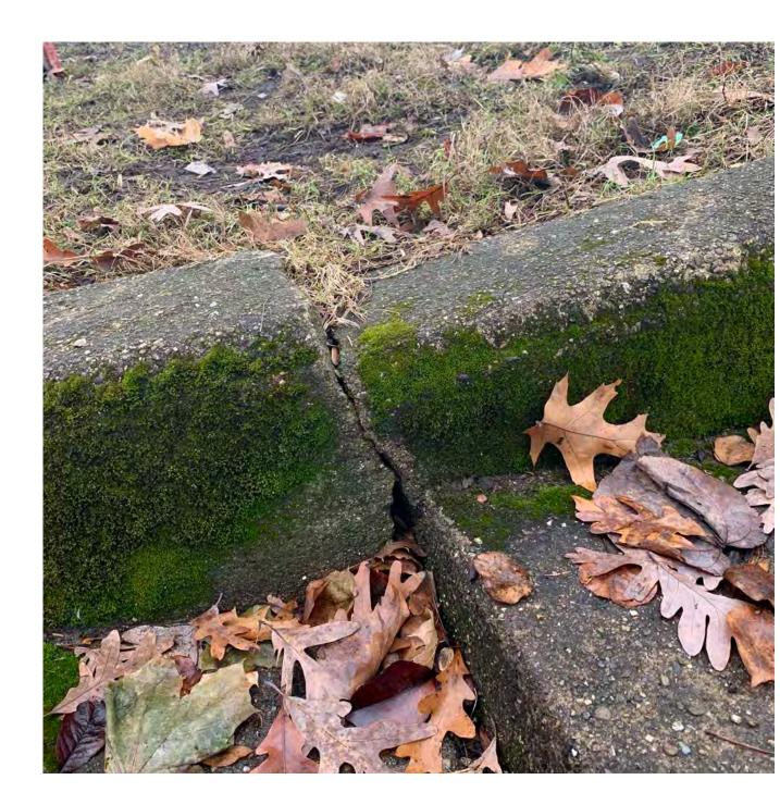
Bottom tier - crack at base of top step continues through wall, entire landing and step has sunk 1"
