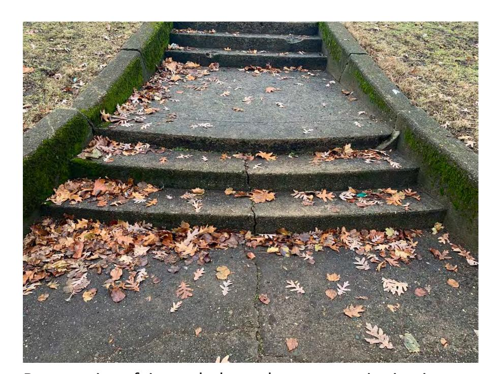
Bottom tier - fair crack through steps continuing into landing, top step 1" lower rise
