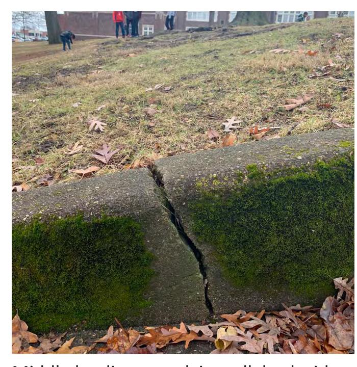
Middle landing - crack in wall, both sides
