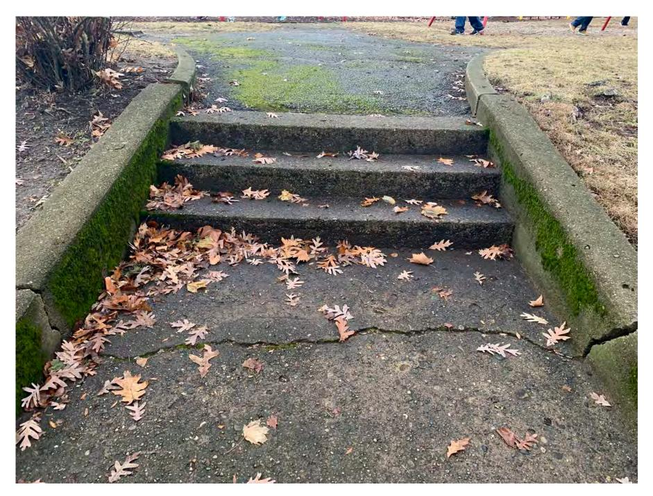
First landing - air condition, significant crack through landing and walls
