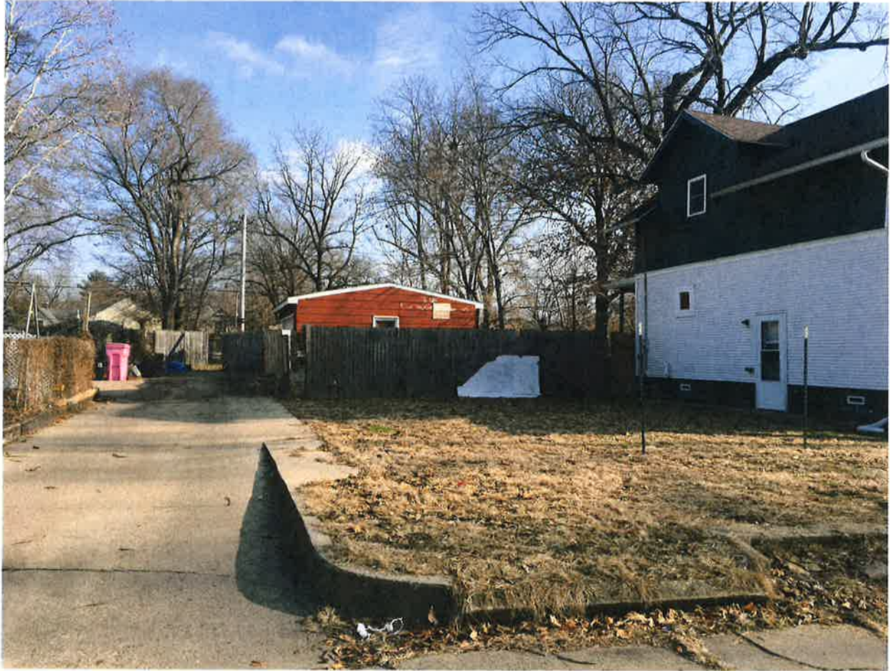
528 N Scott Street Tax ID 018-1055-2336 Vacant, Abandoned, Small Structure See Attached Photos
