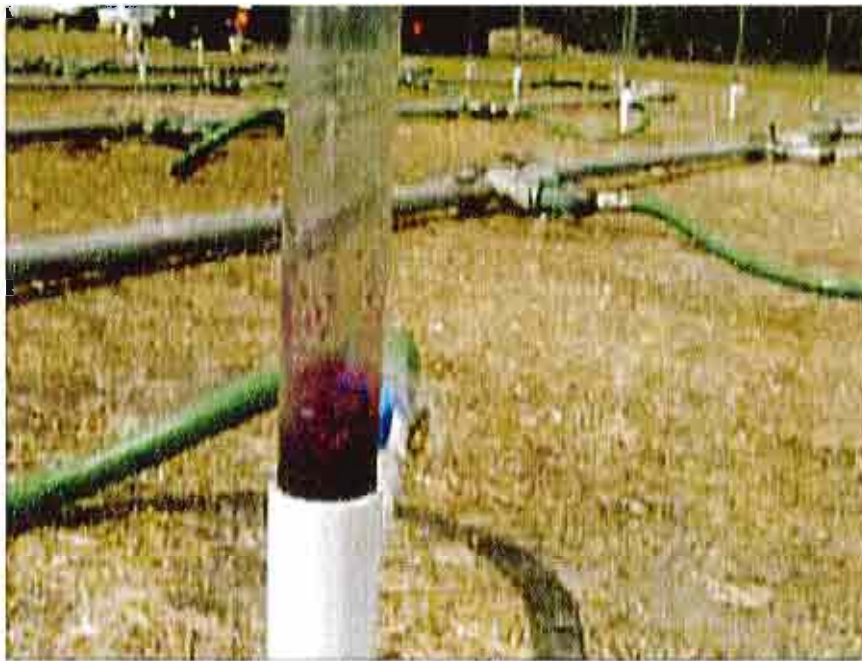
No. 8 – The potassium permanganate solution is being injected.
