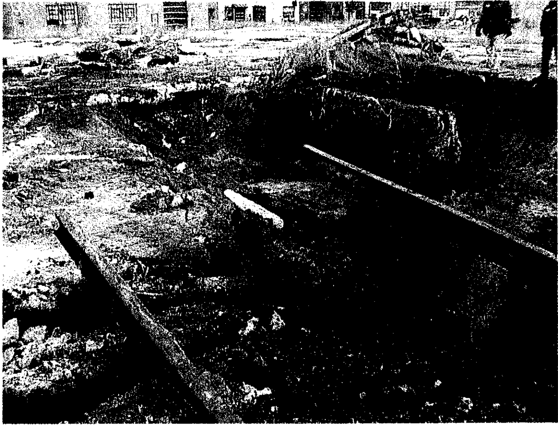
The steel rails and ties of the rail spur are imbedded in the concrete. This view is looking northeast toward the north end of the excavation. One of the concrete monoliths is visible above the rail on the right. The petroleum impacted soil is dark gray and dark grayish brown.
