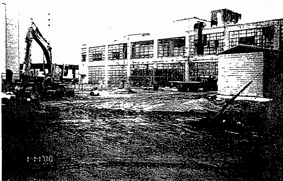
Picture 8: Backfilled Site looking Northwest
