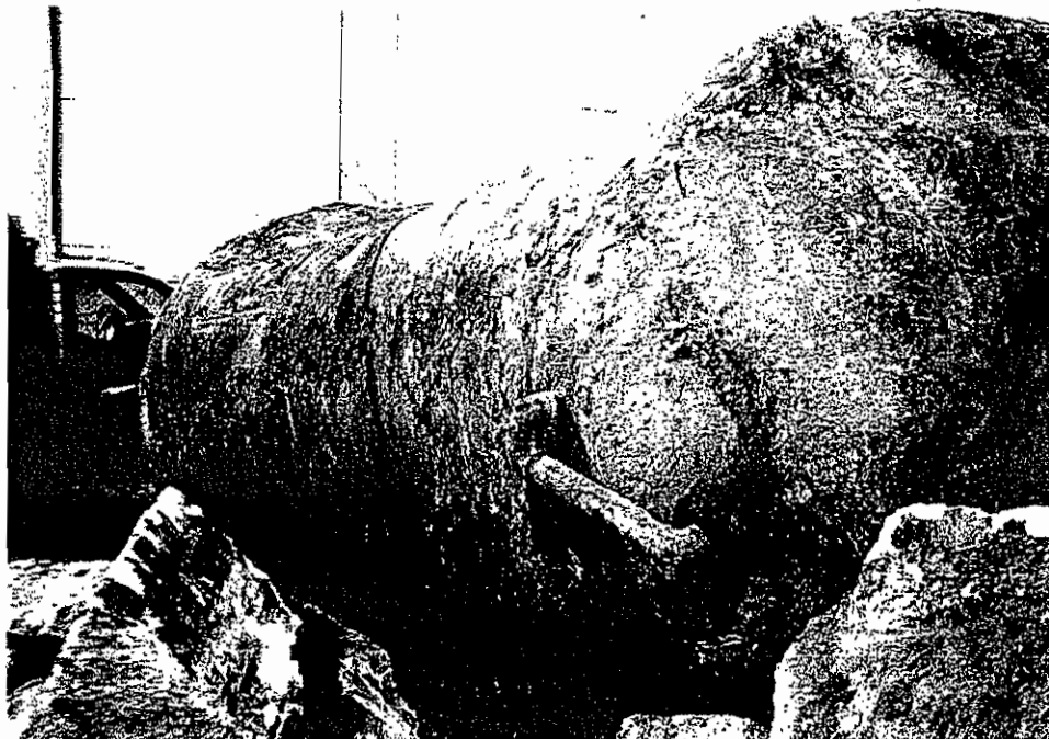
Picture 4: Tank C (note bottom drainpipe connection)
